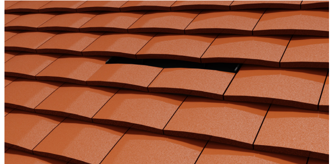
HD TV10/10 Installed
