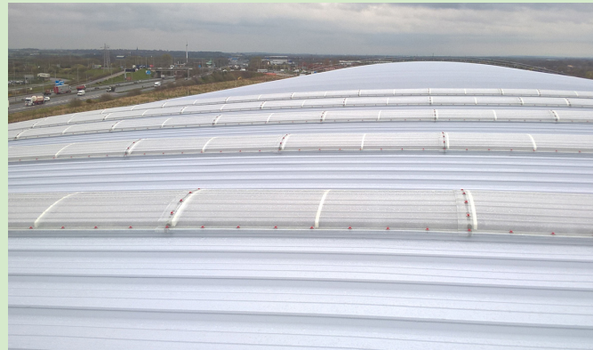
Project: Cornerstone Distribution Centre Location: Warrington Product: Zenon Arc & Pro Liner
