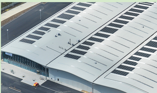
Project: Hitachi Rail Location: Newton Aycliffe Product: Zenon Pro site-assembled Triple Skin
